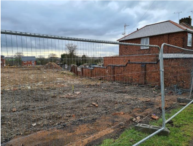
West boundary of site with No:40 Brookhill Leys Road.
